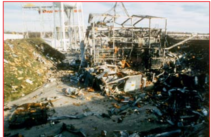
Post-accident debris and damage to rocket motor test facility
